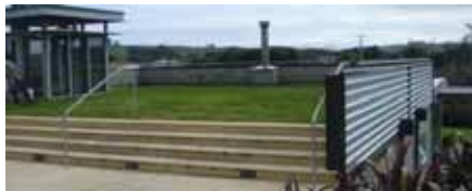
Fig. 5 Beesonline creates recreational space with herbs and lawn species. Selliera radicans would be an alternative species that requires no mowing but would not be as tolerant to foot traffic. Surface water drains to grates that have outlet boxes protruding from the right hand side of the building.
