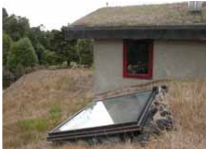
Fig. 6 A sloping greenroof on a domestic dwelling in Canterbury supports pasture grasses, mosses, lichens and native orchids. A skylight protrudes through the lower roof and a chimney through the upper roof.
