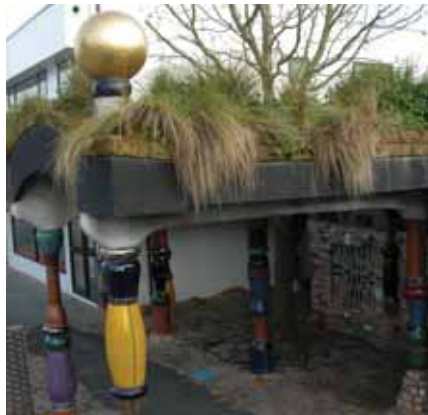
Fig. 2 Kawakawa's Hunterwasser greenroof (front view).
