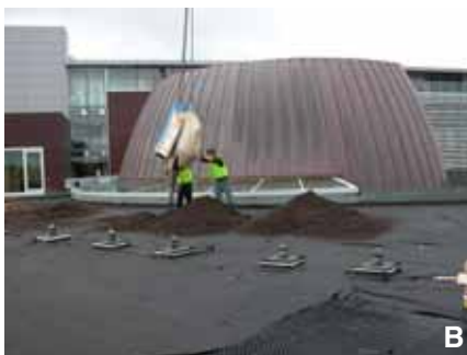
Fig. 9B Substrate must be unloaded without bags resting on the roof (the bags are too heavy). In the foreground interlocking sections of a rigid drainage board can be seen. An overlying filter cloth protects ensures substrate does not block up the drainage board. The Auckland University greenroof used a thinner, lighter, flexible drainage mat with built-in filter fabric. Both drainage materials physically protect the underlying membranes from damage.
