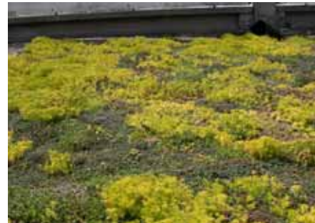
Fig. 8 A sedum mat is rolled out on the University of Auckland roof, creating an instant mosaic of vegetation. The lower photo shows the mat after several weeks.
