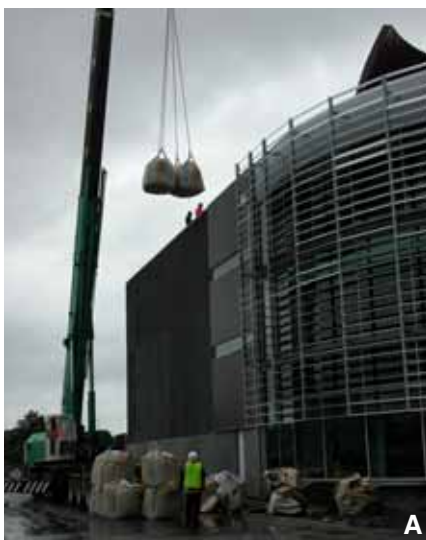
Fig. 9A A crane delivers substrate in bags weighing about 1 tonne each.
