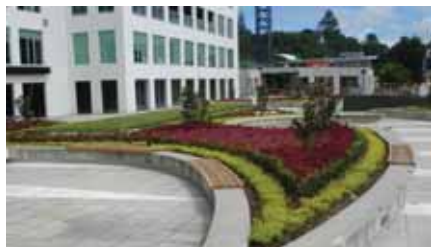
Fig. 1 Intensive greenroof on carpark roof used for amenity and recreational space, Eden Valley commercial building, Auckland.
