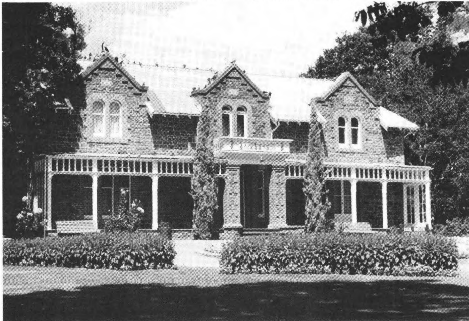
Front of Isel House today. The tree just showing at the left of the house is Magnolia grandiflora ; planted c1865. Now a well-shaped specimen. The two upright conifers on each side of the front door are more recent plantings. The down stairs rooms at the front of the house are administered by the Nelson Provincial Museum and contain china and furniture from the Marsden estate. The upstairs rooms are used by the resident caretaker.
