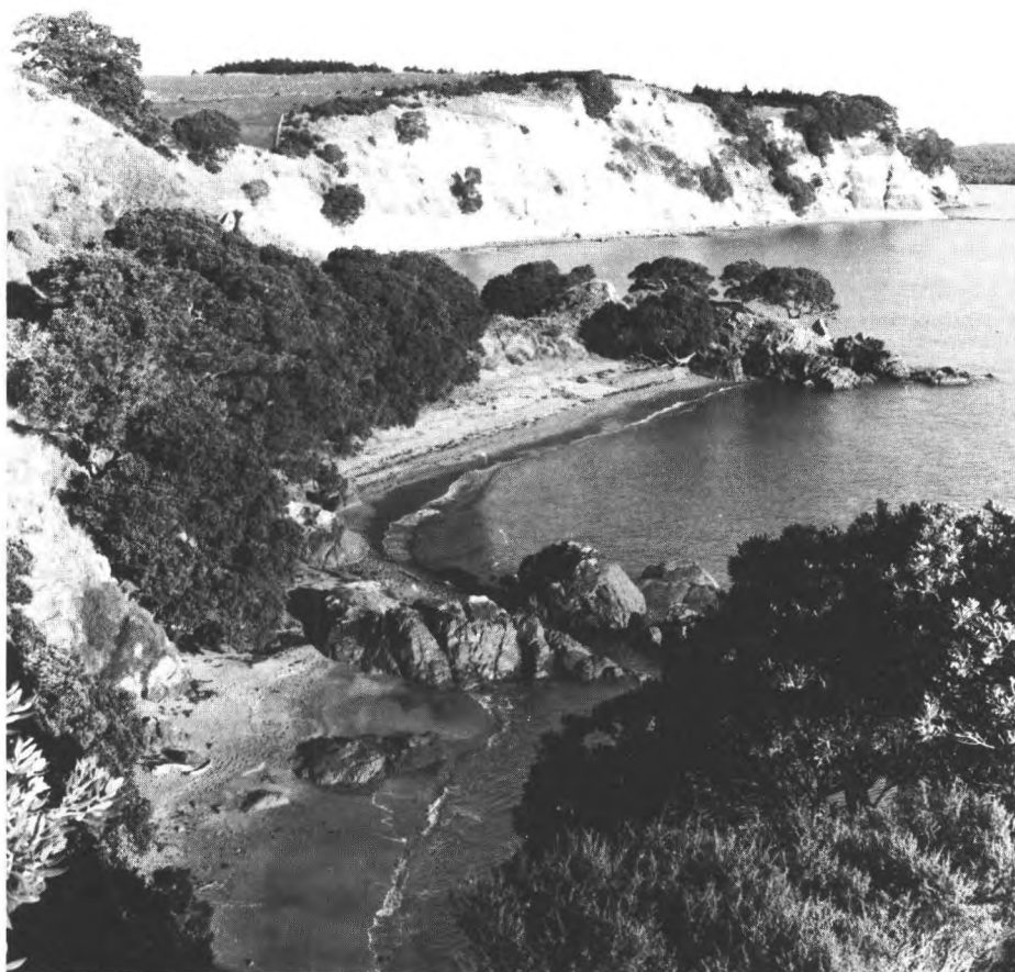
Fig. 3. Motutapu Island: steep, undercut sandstone cliffs with few pohutukawa trees, some of which have slid down from the cliff top. Greywacke in the foreground is stable, gently sloping, and well clothed with pohutukawa trees and grass. (29 November 1977.)
