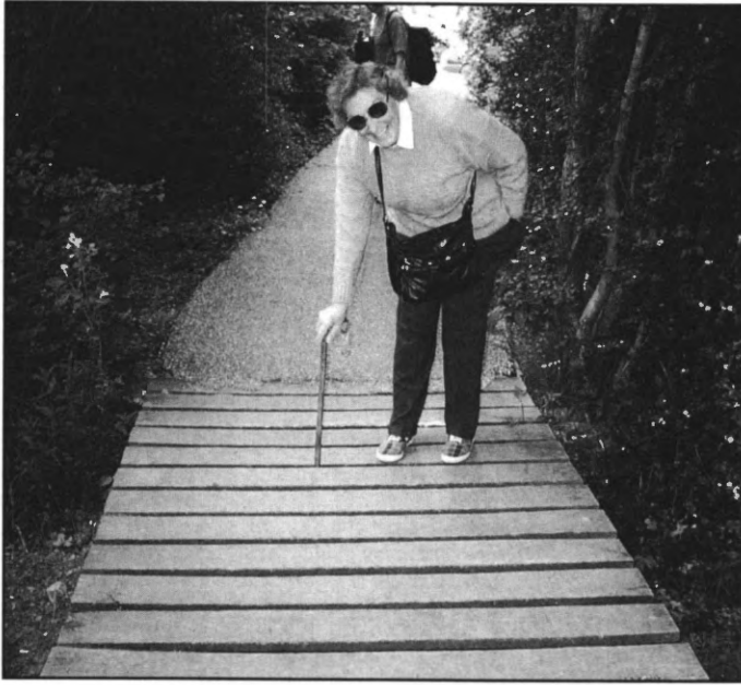
1. Sissinghurst Garden. The main walkway from the carpark to the Garden showing a hazard for people with sticks
