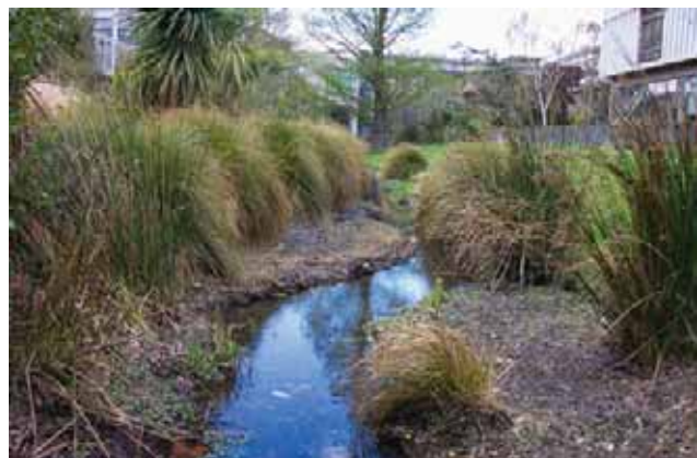
Fig. 9 Sensitive maintenance allowed stream to narrow and a stable channel to form. Meanders have developed and flow is improved. Margin plants can now be planted into reclaimed berms.
