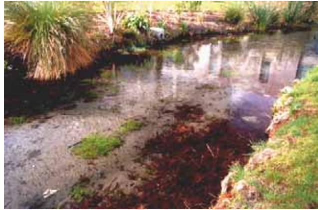
Fig. 5 Silted and over-wide stream bed. The low water velocity allowed silt to smother the stream bed, which reduced the habitat value. Traditional maintenance practices also disturbed the habitat and the removal of vegetation and branches prevented formation of stable in-stream structure.
