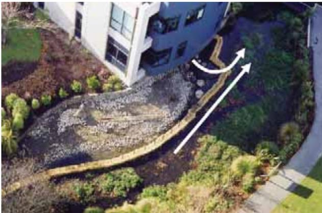
**Fig. 6** Gravel bar constructed to redirect air-conditioning discharge flows and to narrow the stream. Hay bales were used as sediment control during construction. Arrows indicate water flow patterns.
