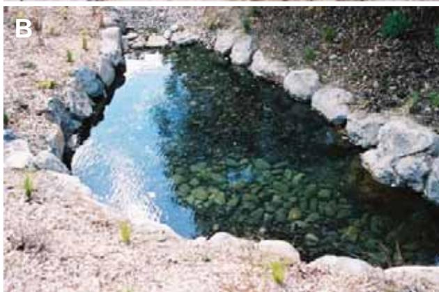
**Fig. 12** Excavation of deep pools provides aquatic refuge when flow stops and also act to trap sediment reducing extent of siltation downstream. **A**, during construction; **B**, completed pools.
