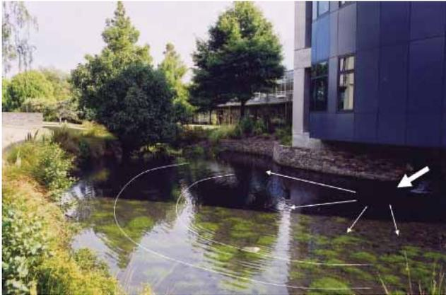
**Fig. 4** Previous flow pattern showing how air-conditioning water discharged from a School of Engineering building impeded flow by pushing water upstream. Photo taken looking upstream. Arrows indicate water flow patterns.
