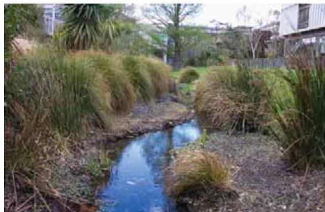
**Fig. 9** Sensitive maintenance allowed stream to narrow and a stable channel to form. Meanders have developed and flow is improved. Margin plants can now be planted into reclaimed berms.
