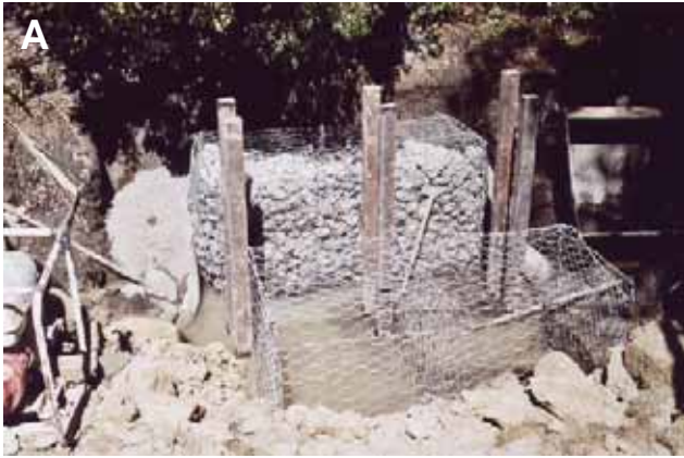
Fig. 13 Special pools designed to provide backwater habitat. Wire baskets of cobbles (gabion baskets) also provide interstitial space and refuge during drying. A , during construction; B , completed pool with backwater habitat at right.
