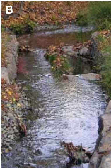
Fig. 13 Special pools designed to provide backwater habitat. Wire baskets of cobbles (gabion baskets) also provide interstitial space and refuge during drying. A , during construction; B , completed pool with backwater habitat at right.
