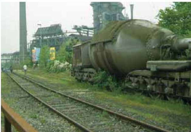
Fig. 1 An industrial park in Duisburg, Germany, with 'riverbed' successions on the railway line and deciduous woodland in the 'ravines' among the buildings.
