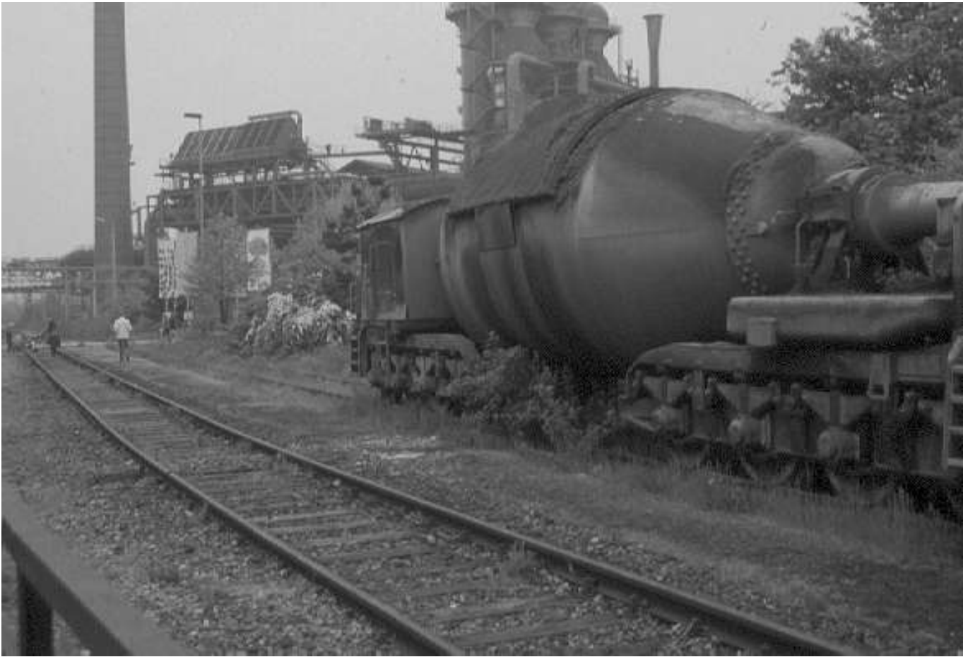
An industrial park in Duisburg, Germany, with 'riverbed' successions on the railway line and deciduous woodland in the 'ravines' among the buildings
