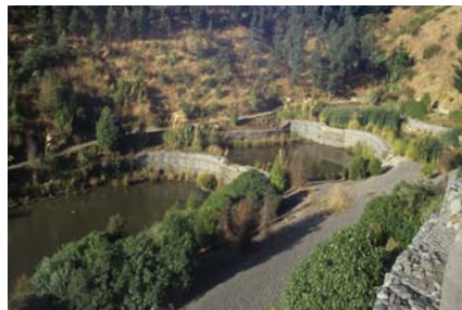
Fig. 20 Cascade of detention ponds on Port Hills, Christchurch with indigenous rushes, sedges, raupo (filter), tussock grasses, shrubs and trees.
