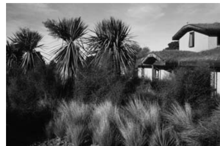
Fig. 3 Green roofs are a way of reducing impacts of rapid stormwater runoff from urban impervious surfaces.
