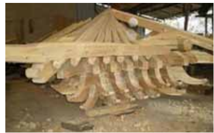
Fig. 9 Hand made roof structure.
