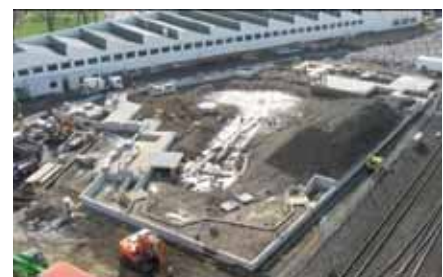
Fig. 15 Overview of site works – the Dunedin input.
