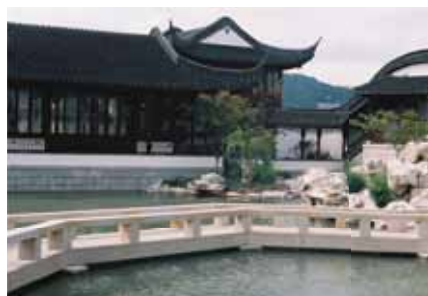
Fig. 18 The newly completed structures.
