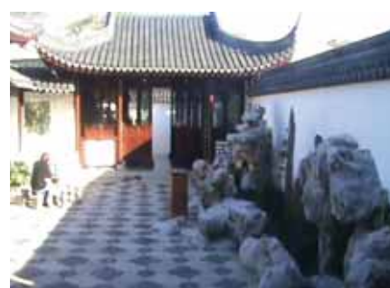
Fig. 5 Northern courtyard and pavilion – note the roof tile detail and the 'swallowtail' roof line. Rainwater is allowed to discharge onto the paving where it is collected into drains and discharged into the drainage system.
