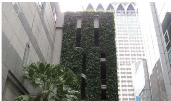
Fig. 4 The six-story high green wall at The Heeren shopping centre.
