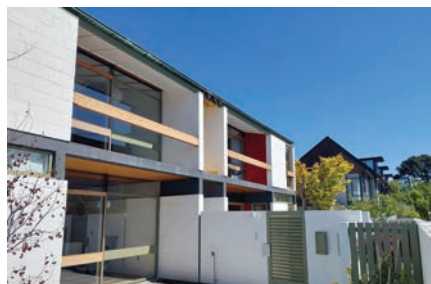
Fig. 2 The Dorset Street Flats, designed by Sir Miles Warren. Photo: Murray Dawson.
