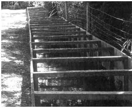
Fig. 2 Papanui Stream before. Boxed drains are waterways that have been confined using timber structures (source: McMurtrie and Walter, 2003).
