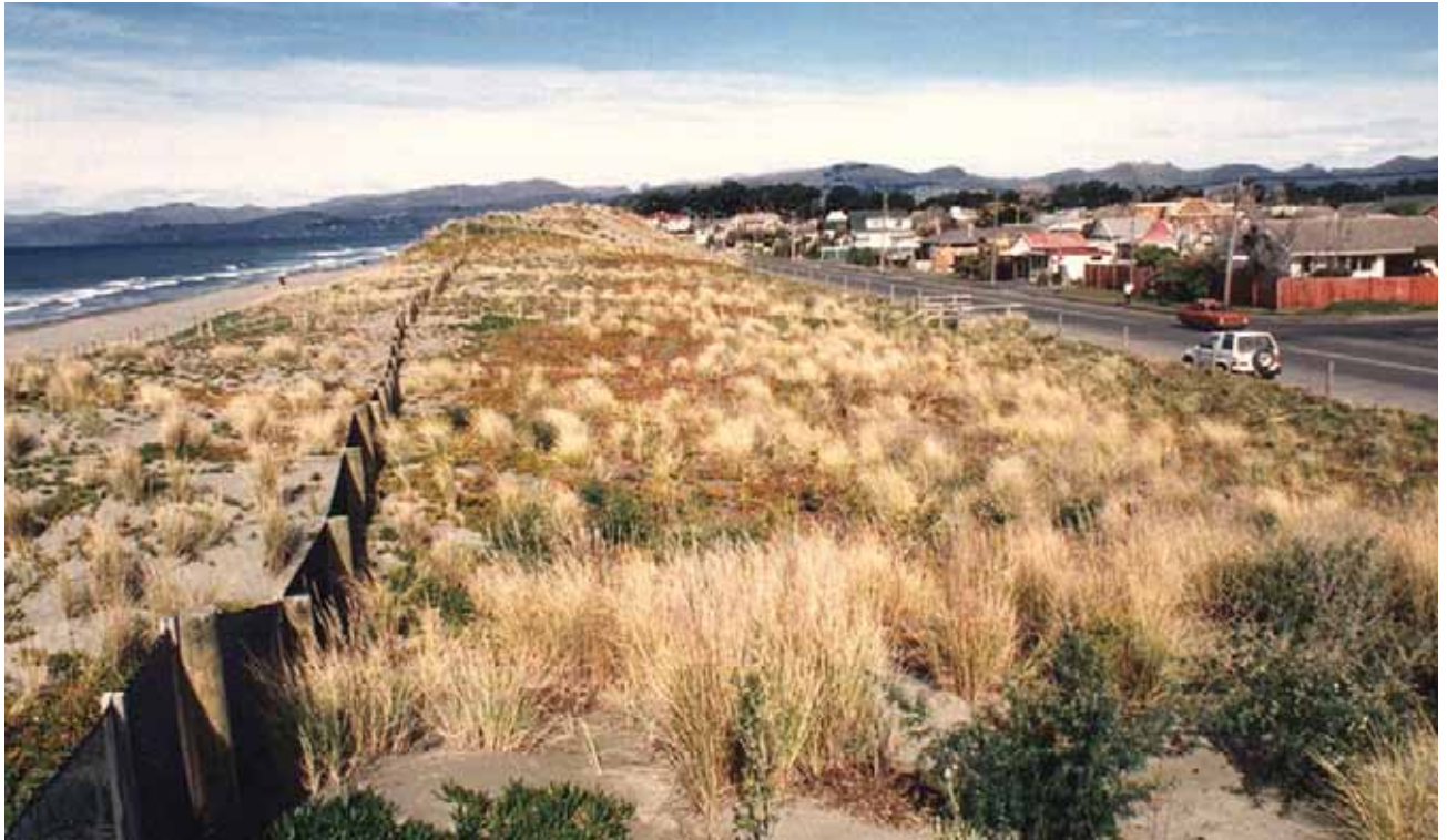
Fig. 1 Dune system adjoining the Christchurch urban area managed primarily for coastal protection. Note the constrained width of the dune, the sand-trap fences and planting for dune stabilisation. (Photo: B. Young).
